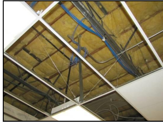
Bracing of suspended ceiling grid
