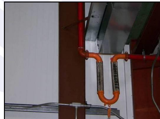
Flexible coupling for piping
