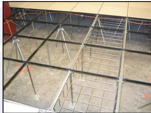
Raised-access floor bracing system
