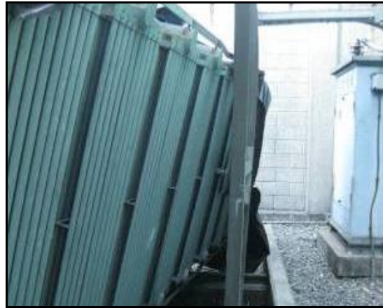
Transformer damage can lead to prolonged downtime (2010 M8.8 Chile earthquake)
