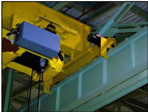
Bridge crane vertical restraint
