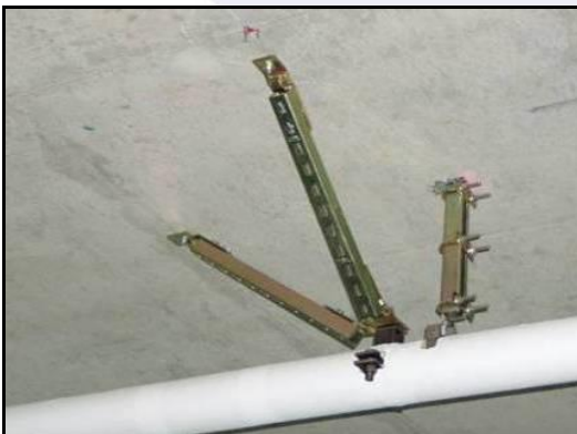
Lateral and vertical bracing for piping
